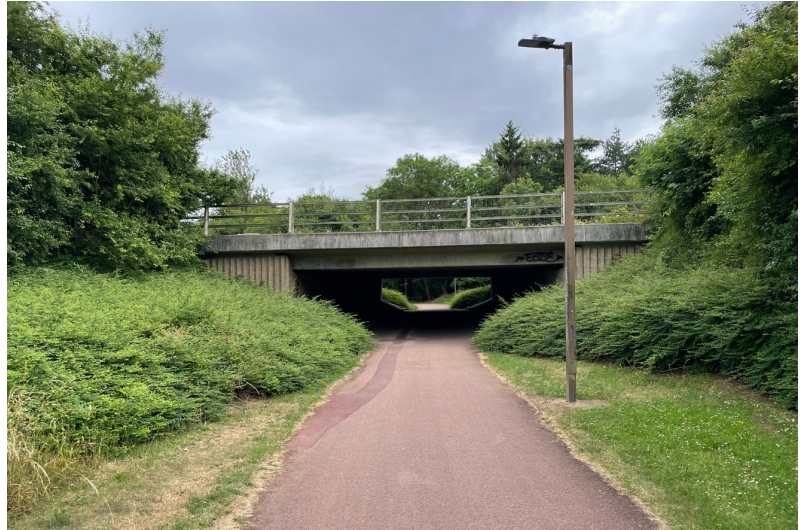
Figure 49: Example underpass in MK (lit, direct and through visibility evident)
